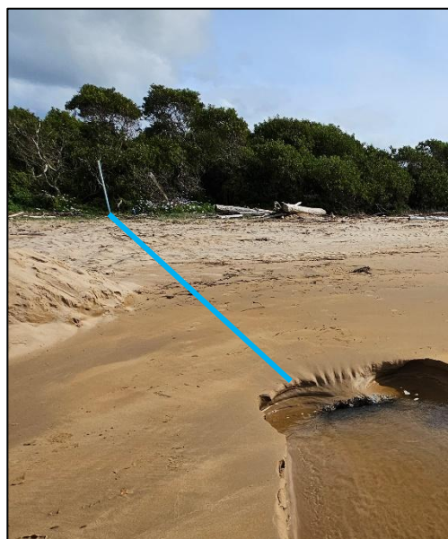
Figure 4: Looking inland from the old storm drain that will be replaced to the blue pole that shows the start of the proposed works.
