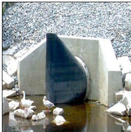
Figure 7: Duck bill flap over storm drain
