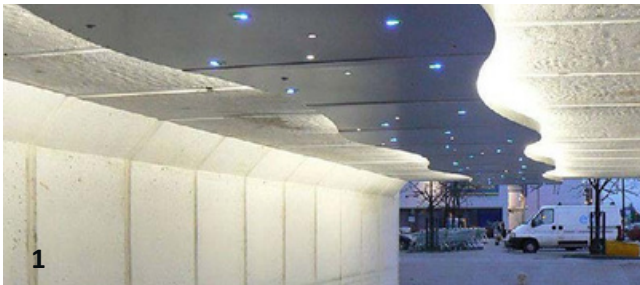
Light installation with Leven River design fixed to roof with pinpoints of light reflecting on concrete wall and floor.
