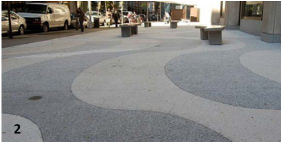
Contrasting bands of concrete paving with Leven River design on footpath leading into Laneway, creating continuity between ground plane and roof motif.
