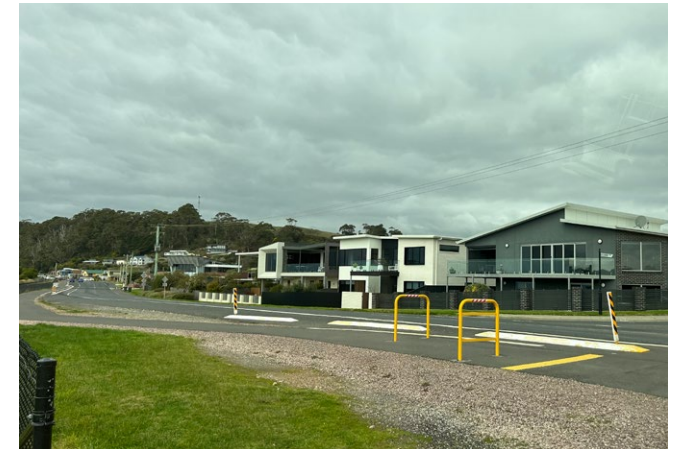
45 Sulphur Creek foreshore facing development
