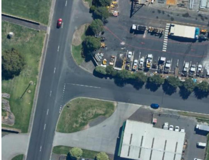
Figure 11 – Aerial view of Fieldings Way / Industrial Drive junction
