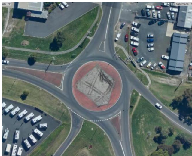
Figure 7 – Aerial view of Eastland Drive / Fieldings Way Roundabout
