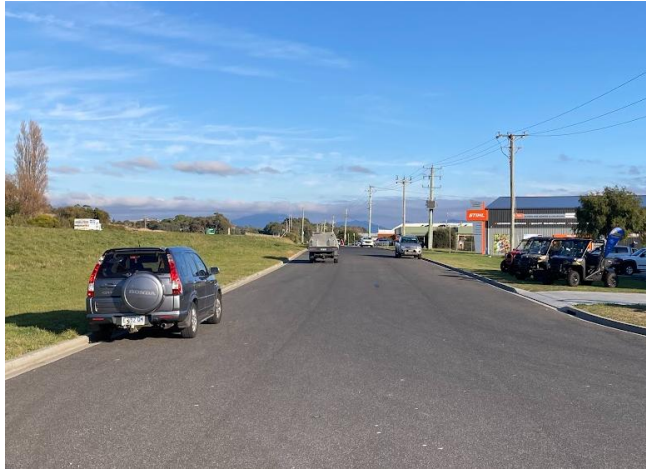
Figure 22 – West bound on Industrial Drive from extension site
