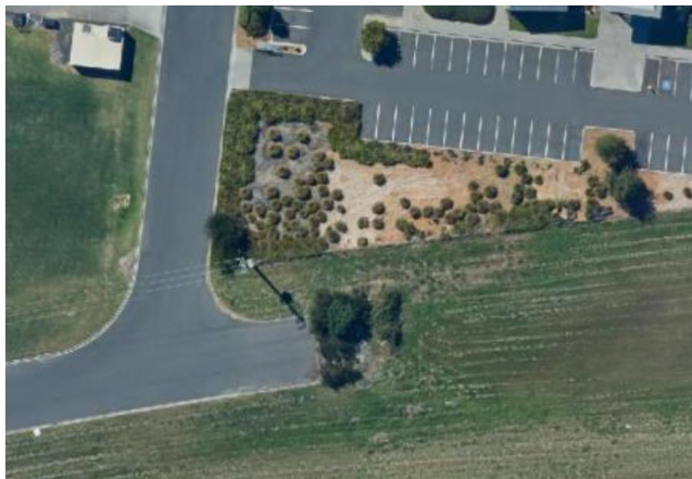
Figure 17 – Aerial view of proposed Industrial Drive extension site
