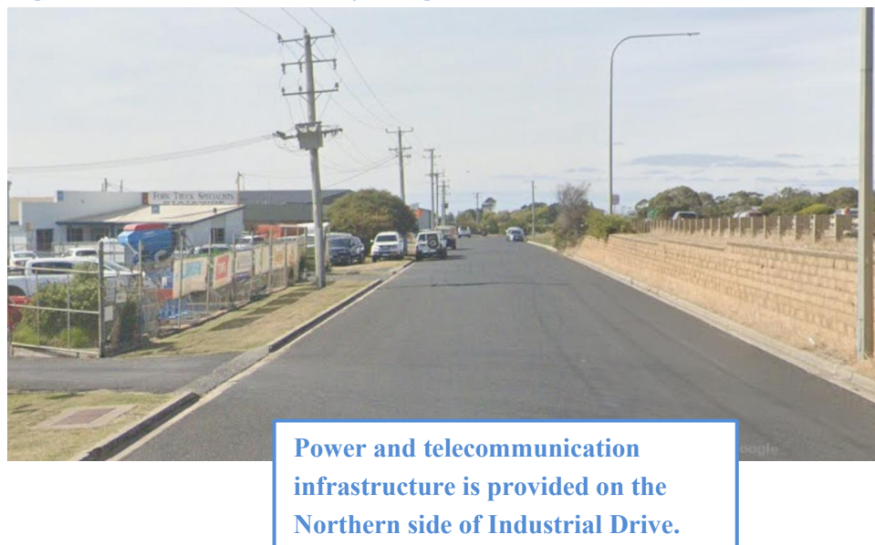
Figure 37 – Eastbound midway along Industrial Drive
