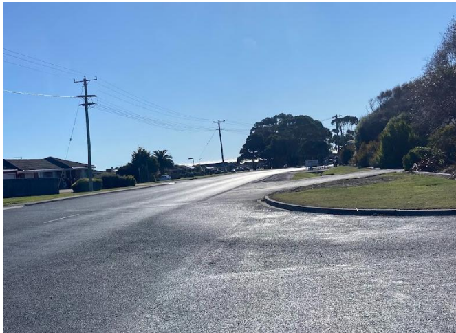
Figure 14 – Looking right along Fieldings Way from Industrial Drive
